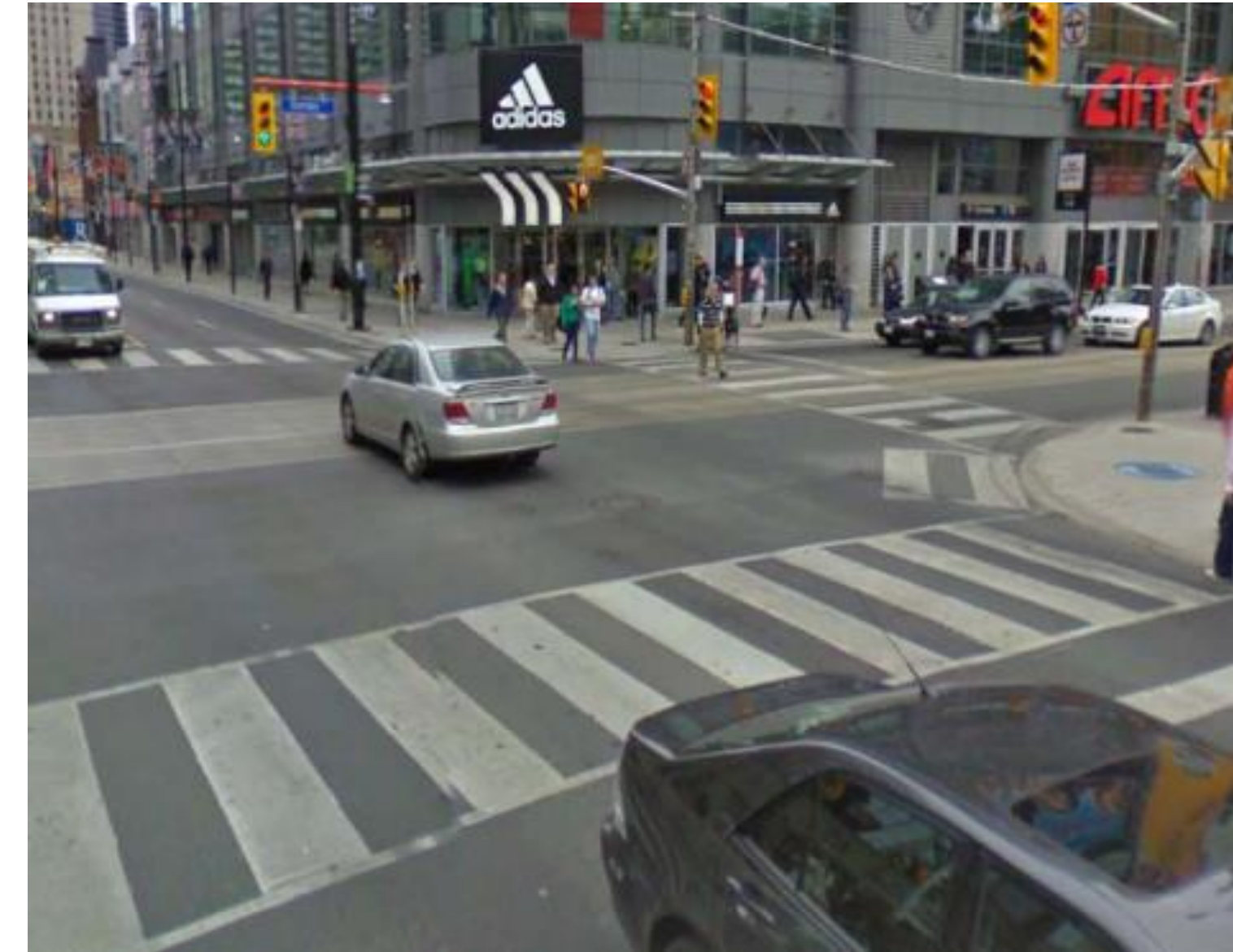
Enhanced crosswalk marking
