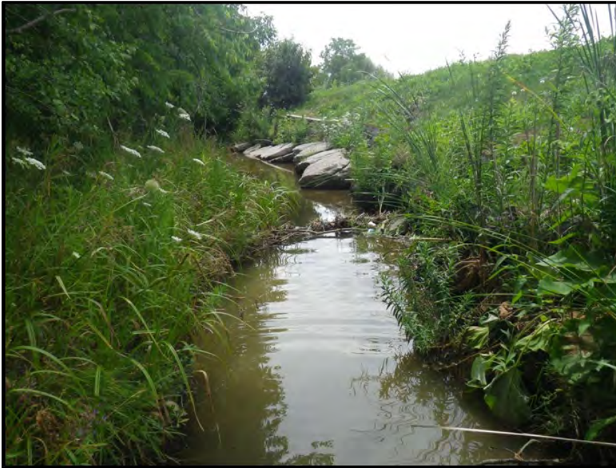
31. Reach C-7: ponding upstream from armourstone bank protection
