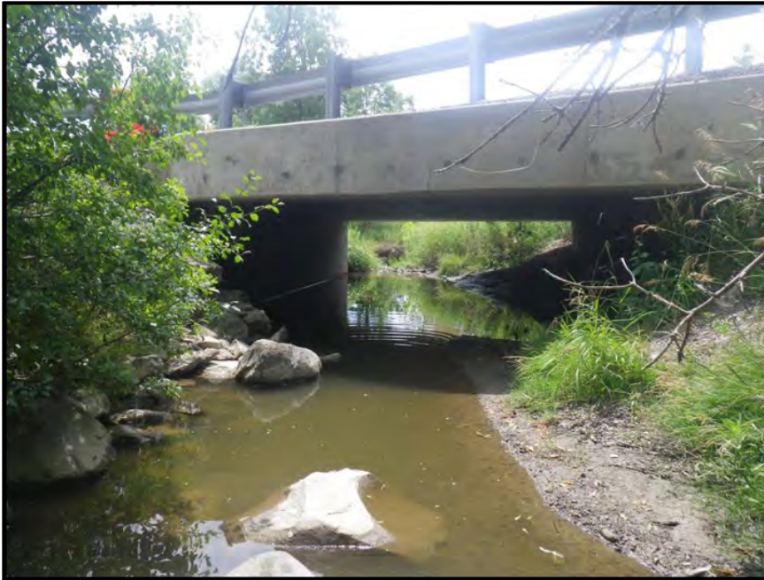
33. Reach C-7: crossing at Clarkway Drive; south bank protected by boulder placement
