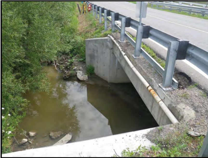
39. Reach C-8: view of Countryside Drive crossing from Clarkway Drive; approach angle of channel causes erosion and scour
