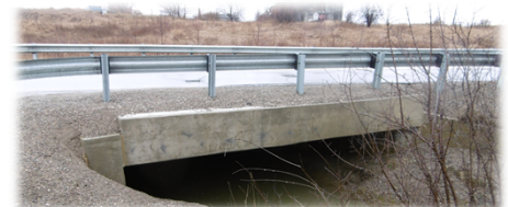
Clarkway Drive over Clarkway Tributary
