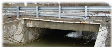
Countryside Drive over Clarkway Tributary
