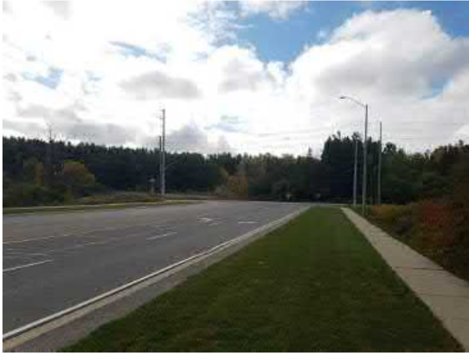
Photograph No. 3 – South-facing view of the Site, depicting Countryside Drive.
