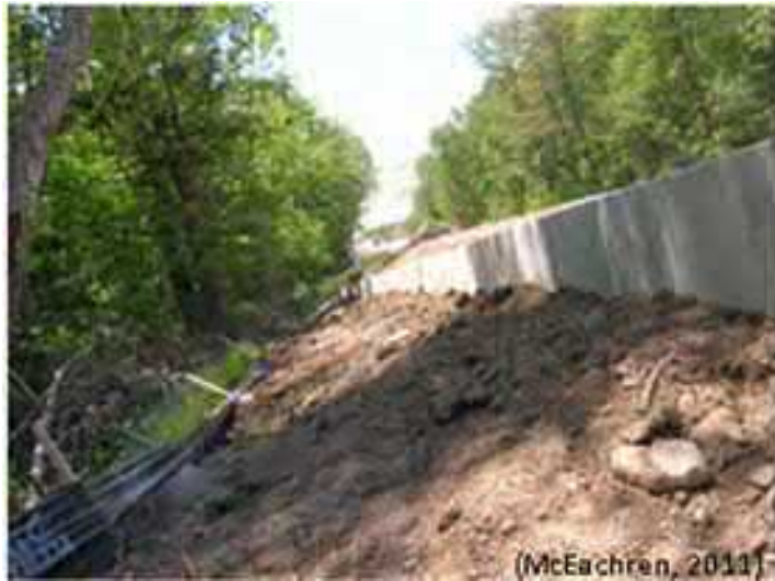
Image 6: Permanent Concrete Wall Directing Wildlife to Underpass
