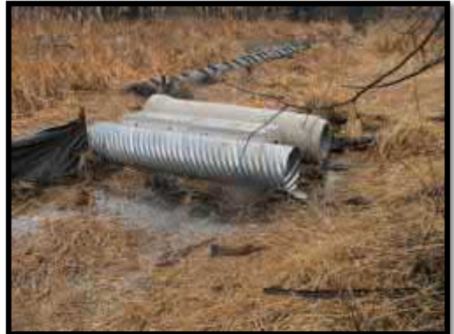
Figure 10 – Textile fabric at culverts
