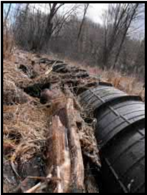
Figure 5 – ACO fence banked material
