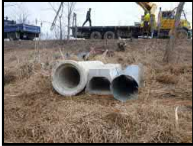
Figure 8 – Culverts in place
