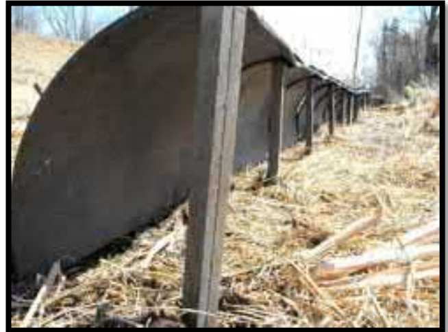
Figure 4 – Inside edge of ACO directional fence
