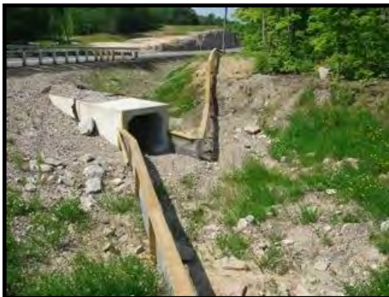
Figure 60. Oversized concrete box culvert.
