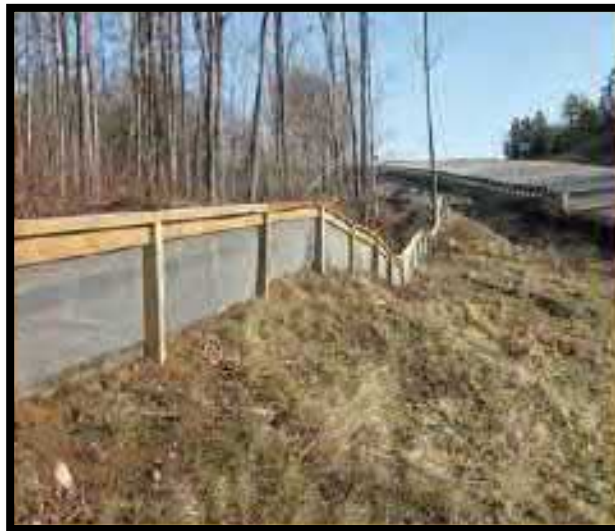
Figure 67. Directional fencing, partially buried hardware cloth fence with rail (MNR, 2013).
