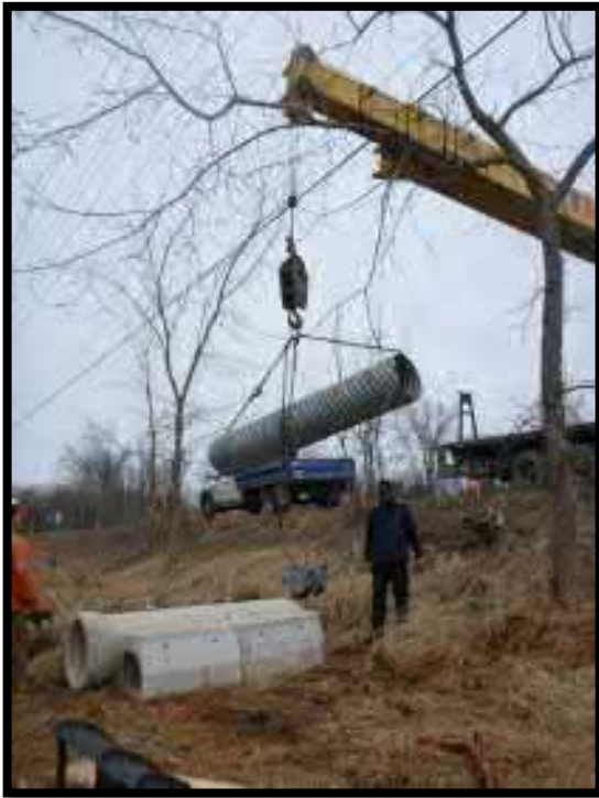
Figure 7 – Crane positioning culverts
