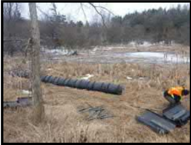
Figure 3 –Staff installing ACO directional fence
