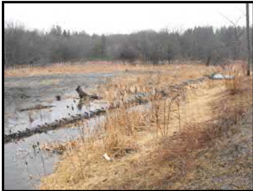
Figure 15 – Mock culverts and ACO wildlife directional fencing in place
