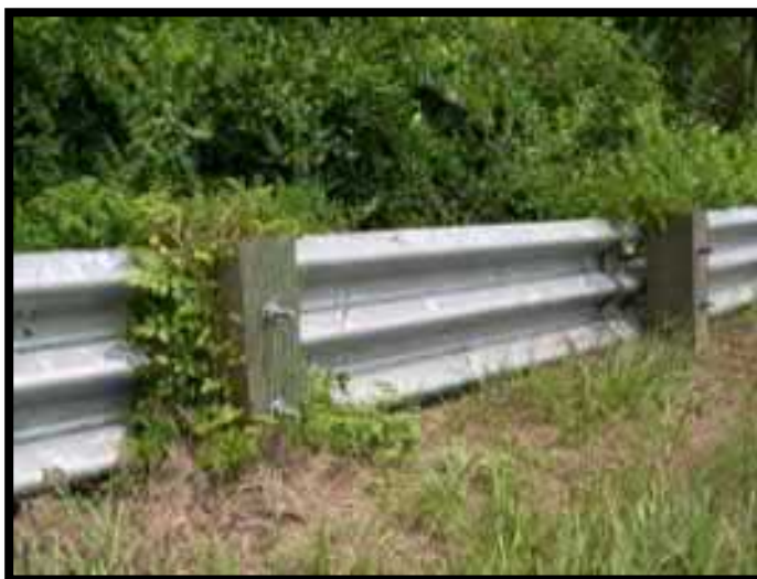
Figure 64. Directional wildlife fence, buried guardrail (Photo Credit: Aresco MJ).
