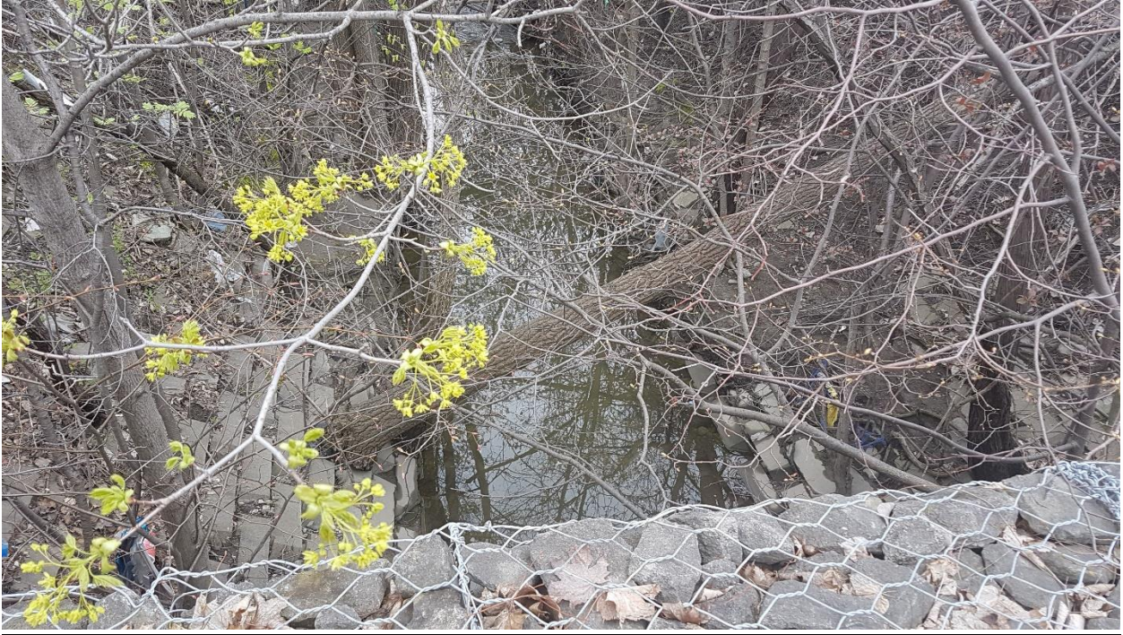
West boulevard at Hansen Road looking east downstream of crossing
