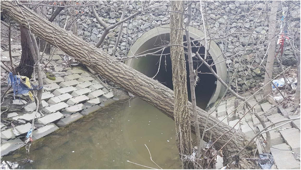
West boulevard at Hansen Road looking west at culvert
