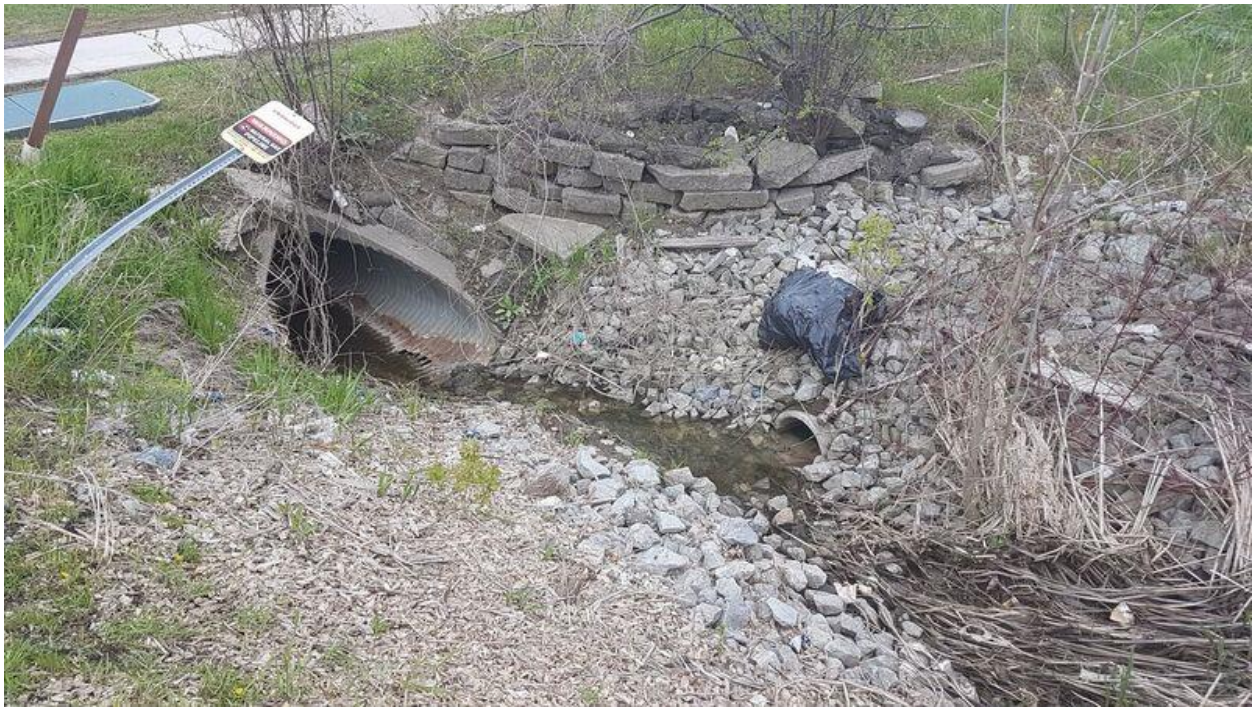
West boulevard at Hansen Road looking east at culvert
