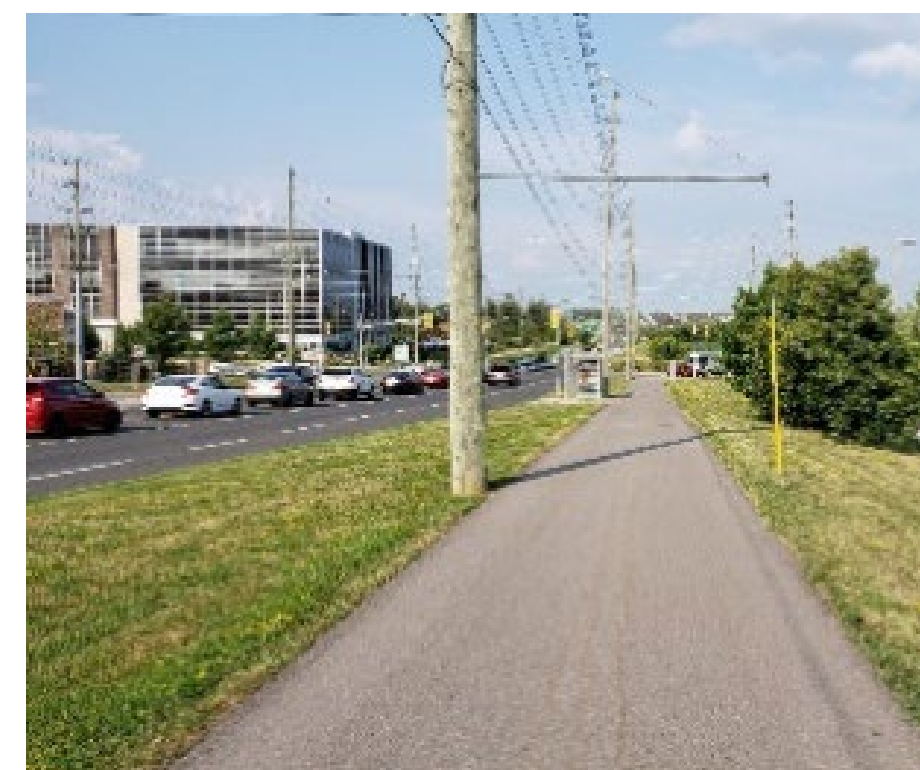
Multi-Use Path Pedestrian and cyclists share space in boulevard
