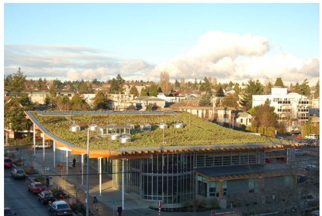
Green Roofs regulate building temperatures, decrease energy consumption and reduce stormwater runoff - Ballard Library in Seattle, Washington
