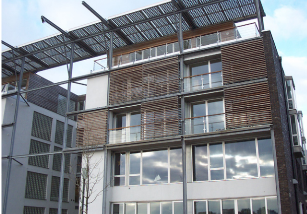
Heat gains in warmer months can be minimized through building design – Malmö, Sweden
