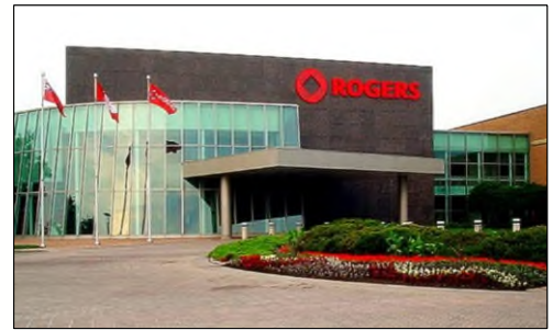
Figure 11: Rogers Communications Corporate Campus, a 25-ha (62 acre) site is one of Brampton's largest non-industrial employers in an Employment Area.
