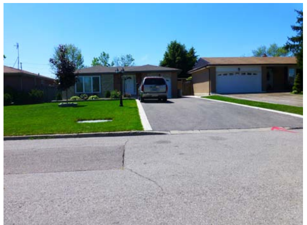
Example of a typical bungalow with larger front and side yards in Neighbourhood 4
