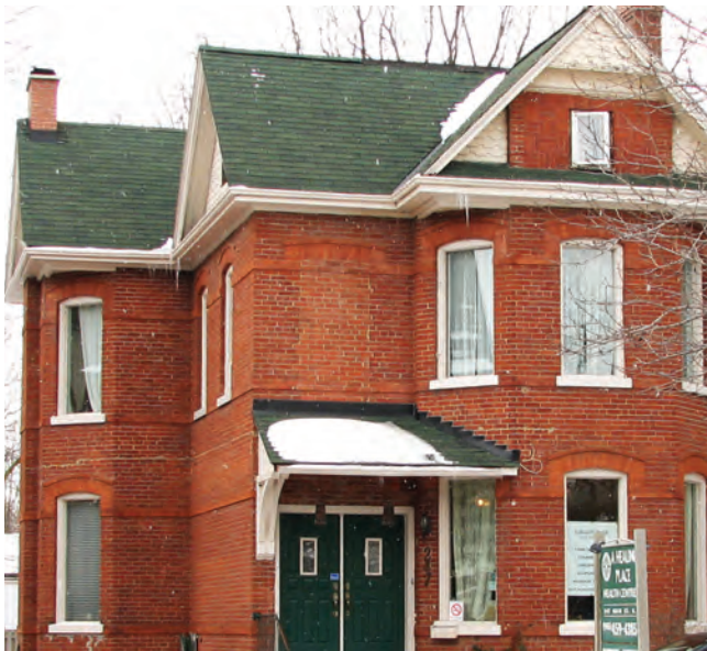
Figure 6-10: The Heritage Value of This Building Has Been Diminished by Inappropriate Plate Glass Thermal Windows
