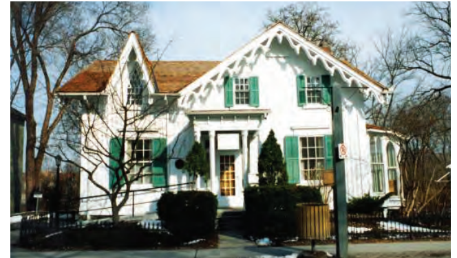
Figure 6-13: Inappropriate Access Ramp Location & Design
